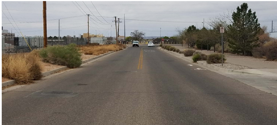
FIGURE IIIB.3. INNOVATION PARKWAY IPOC EAST DRIVEWAY TO SOUTH EUBANK BLVD. TYPICAL SECTION
