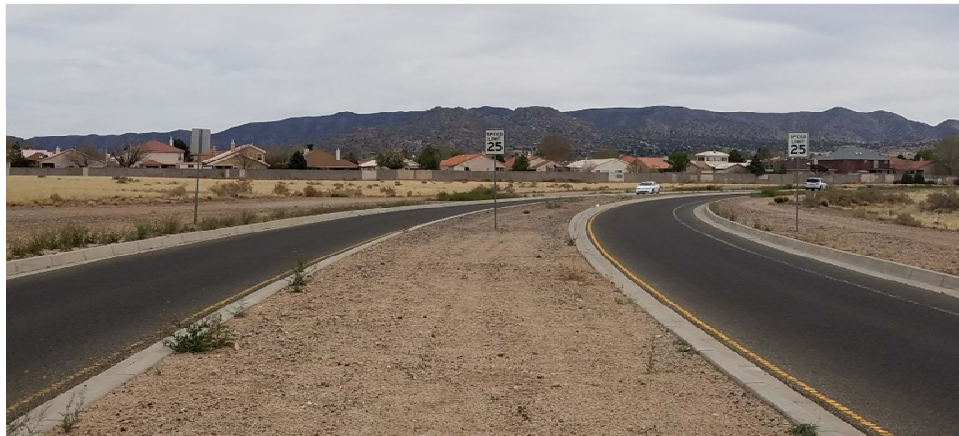
FIGURE IIIB.1. INNOVATION PKY. NORTH EUBANK BLVD. TO SOUTH OF RESEARCH RD. TYPICAL SECTION
